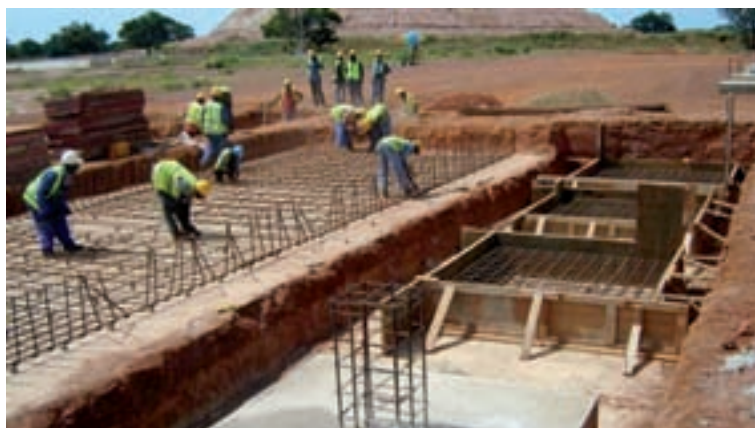
Foundations being prepared for Blackthorn Resources' Perkoa processing plant
